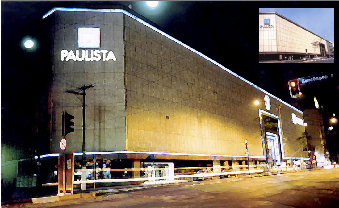
The Paulista mall is controlled around the clock by an InduSoft building automation system.
