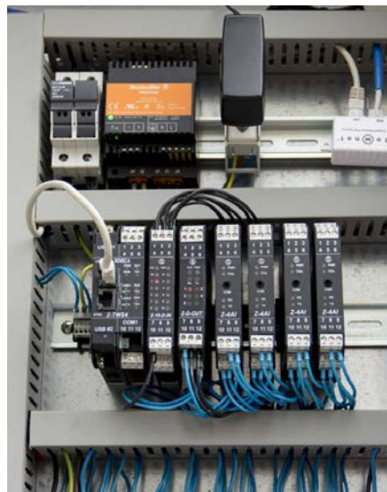
Peripheral unit panel detail
